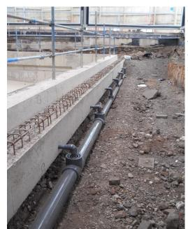
Over time with the lack of support the pipework eventually gave way.
