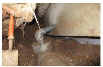
The structural Engineer's design was for the filtration pipework to be supported with reinforced hangers from the suspended ground floor slab at 1.5m c/s.
