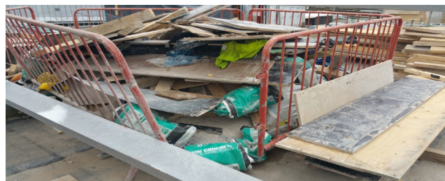
This photo depicts a lack of respect for the hotmelt covering.
