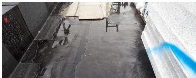
This photo shows the voids and undulation surface finishes which become damaged and allows water ingress.
