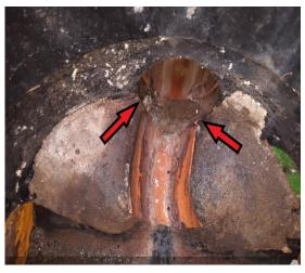
We rectified the issue using a 150mm clay radius channel connecting the inspection chambers inlet and outlet as 1 continuous run, this reduced the chance of debris build up and aided the foul waste to run through the chamber as expected.
