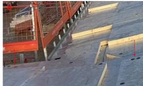
This is compounded further by the installation of the second board layer, when laid in to a large area prior to fixing the profile location is not clear unless setting out has been conducted to pinpoint the location, this results in the VCL being punctured several times, until the top of the profile is found. Interim inspection and HOLD points
